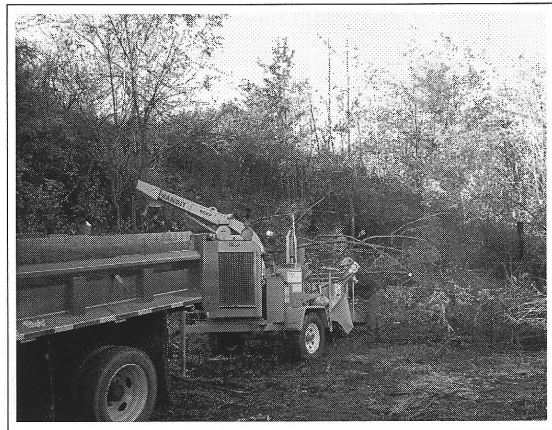
Town Highway employees chipping the brush on the connection
